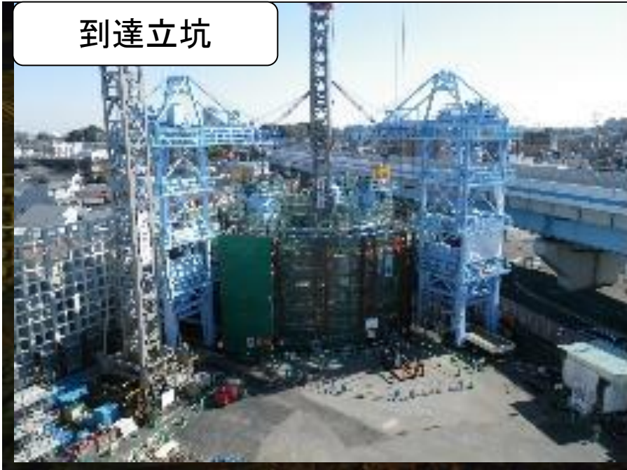
Excavation at Arrival shaft
