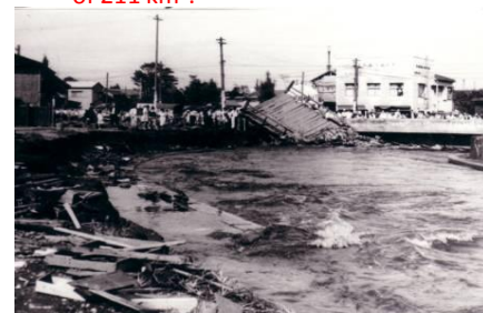
Flooding along Shakujiigawa River
