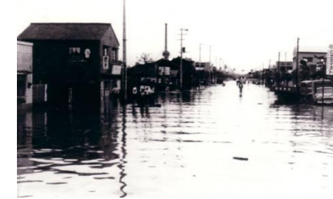
Flooding along Nakagawa River
