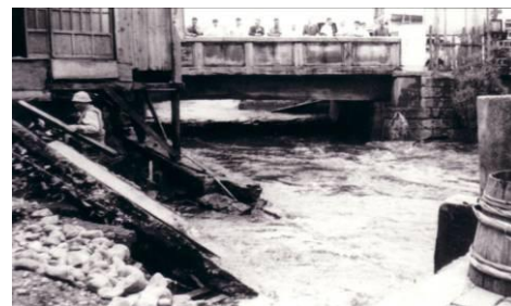
Levee breach around Taishibashi Bridge over Karasuyamagawa River in Taishido, Setagaya Ward
