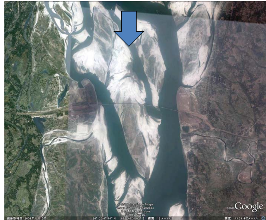
Jamuna Bridge in Bangladesh
